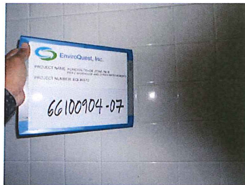
Photo #10: Ground floor, restroom. Non-asbestos containing white ceramic wall tile and grout.
