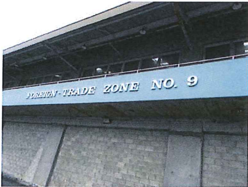
Photo #1: Foreign Trade Zone No.9 Pier 2 warehouse.
