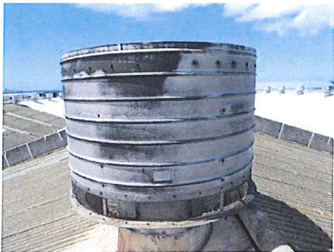
Photo #50: Roof. Non-lead based painted silver exhaust fan.
