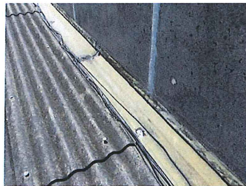
Photo #34: Roof flashing. Non-asbestos containing black and white caulking.
