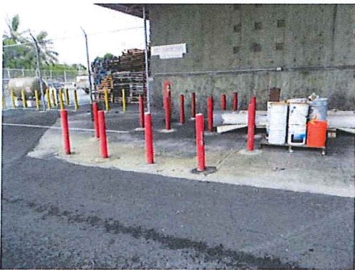
Photo #54: Non-lead based painted red bollards.
