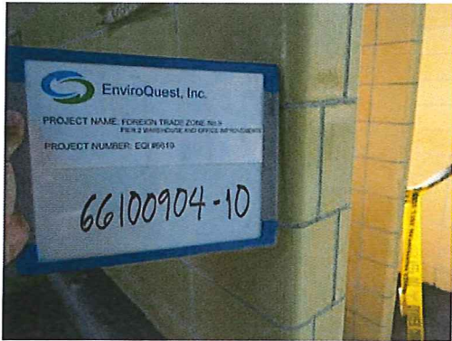
Photo #13: 2nd floor, urinal area. Non-asbestos containing beige ceramic wall tile and grout.
