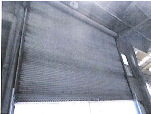
Photo #46: Ground floor. Non-lead based painted light-green roll-up door.
