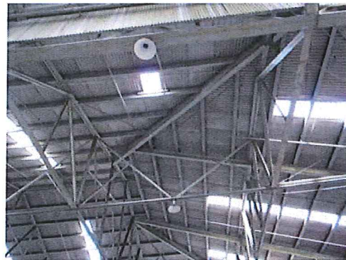
Photo #51: Roof trusses: Lead-based painted light-gray metal trusses.
