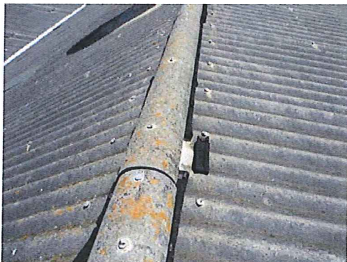
Photo #23: Roof ridge. Non-asbestos containing black sealant. Asbestos-containing cementitious roof and ridge.
