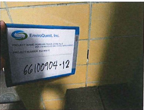
Photo #15: 2nd floor, shower room. Non-asbestos containing beige ceramic wall tile and grout.
