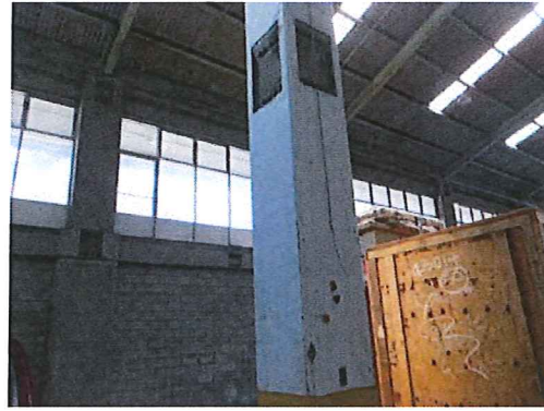
Photo #38: Ground floor. Non-lead based painted white concrete column (upper portion).
