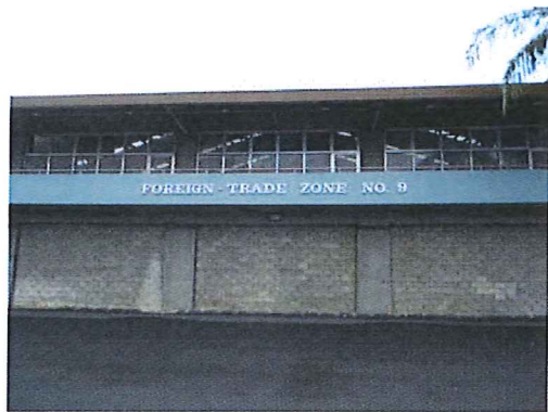
Photo #56: Non-lead based painted gray canopy exterior wall.
