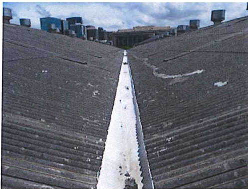
Photo #35: Roof gutter. Asbestos-containing roofing felt under non-asbestos containing elastomeric coating and tar.
