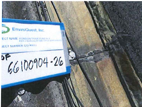
Photo #31: Roof flashing. Non-asbestos containing black and white caulking.
