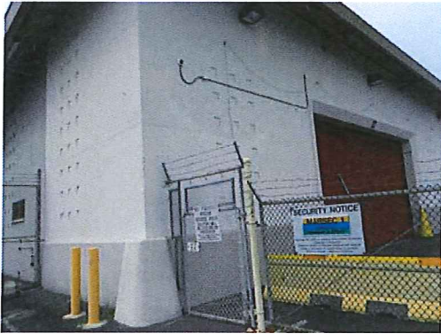
Photo #52: Non-lead based painted off-white exterior wall.
