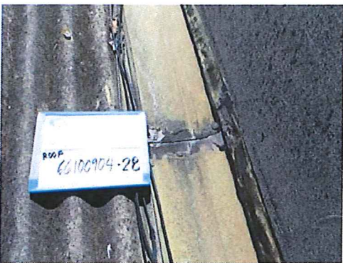
Photo #33: Roof flashing. Non-asbestos containing black and white caulking.
