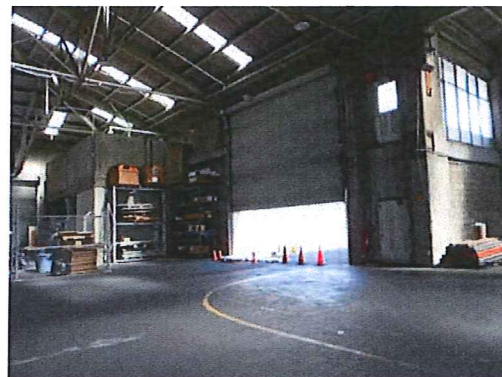
Photo #6: Ground floor. Non-asbestos containing black flooring (asphalt).
